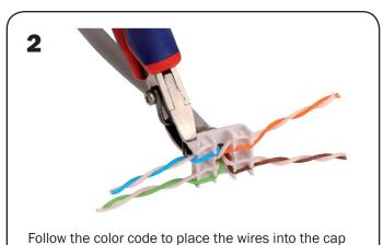
slots. Keep the pairs twisted as possible and cut of
